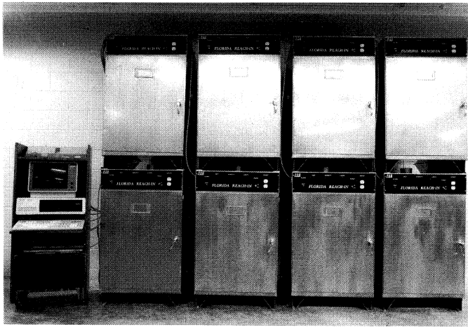
Fig. 1. Eight Florida Reach-Ins. Control and logging are by computer at left.
